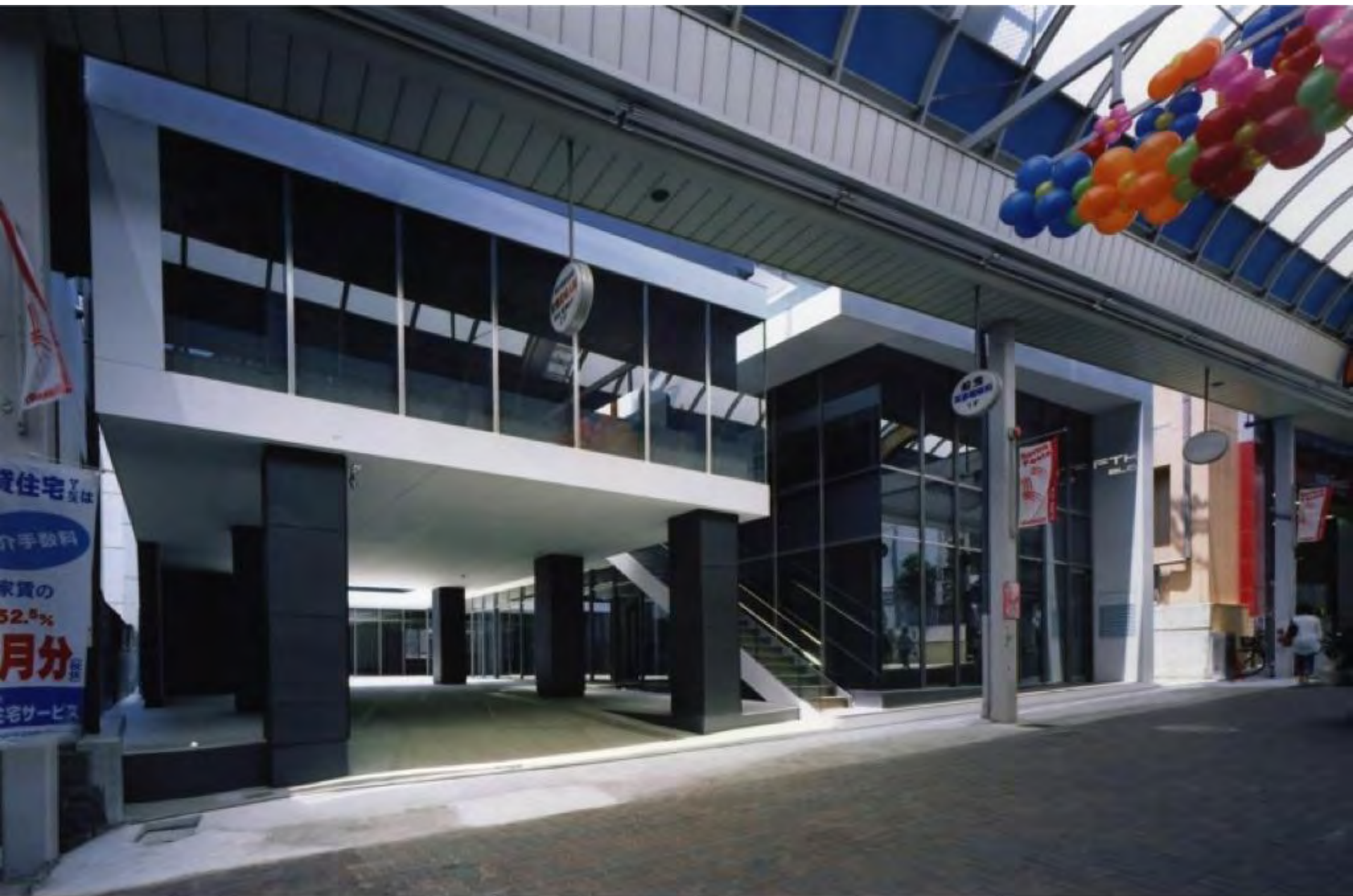
FTK Building after Refining
