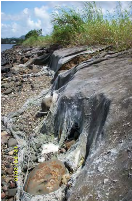
Picture 16 Bottom left – Coastal erosion along Baro subdivision foreshore, eroding rock revetment wall containing loose and fraying geo-textile material.
