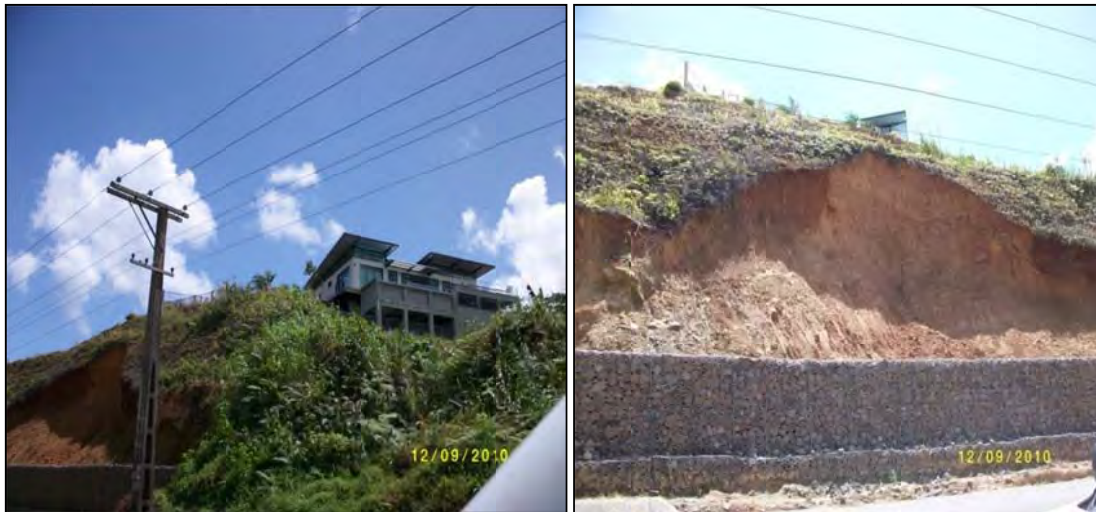
Pictures 6 & 7 Continually sliding area of land with rock revetment wall at entrance to Panoramic Road
