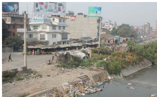
Waste along the river, close to the community market Photo © Ilija Gubic
