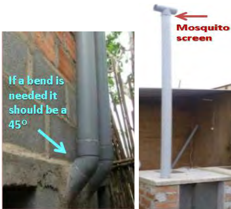
Figure 14: Ventilation pipe with 45° bend, mosquito screen and T-tubing (Rotaria, Peru).
