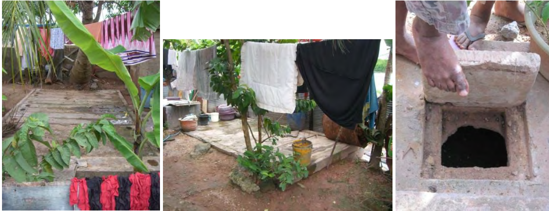
Figure 4: Septic tanks in gardens with opening for gully suckers
