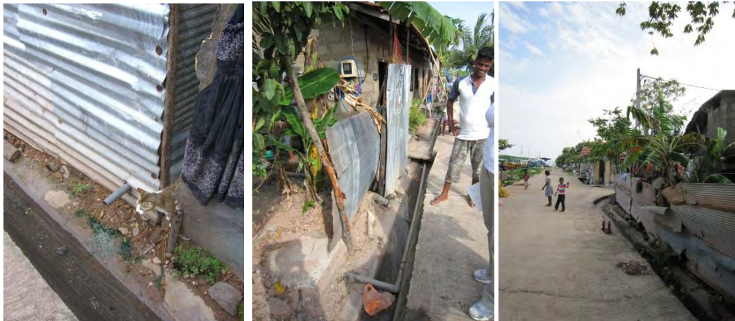
Figure 5: Open drainage of grey water at Monako Gama
