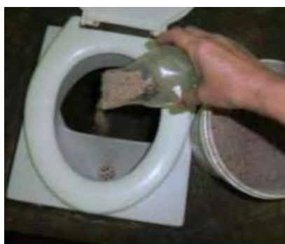
Figure 13: Adding of dry material after toilet use. Dry material is stored in bucket with plastic cup next to toilet (Rotaria, Peru).
