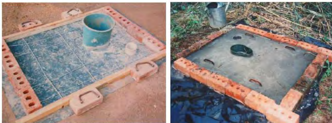
Figure 11: Different stages when toilet floor is made (Fotos Peter Morgan)
