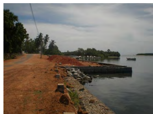
Gabion walls built to control flooding
